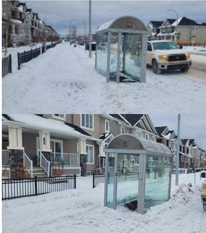
Heritage Drive: There is about 6-8 inches slope difference from the sidewalk to the curb
