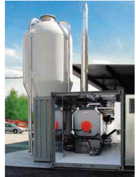
Portable boiler enclosure (pellet silo field supplied)
