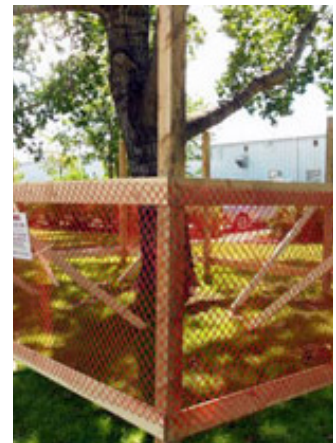
Example of tree protection during construction
