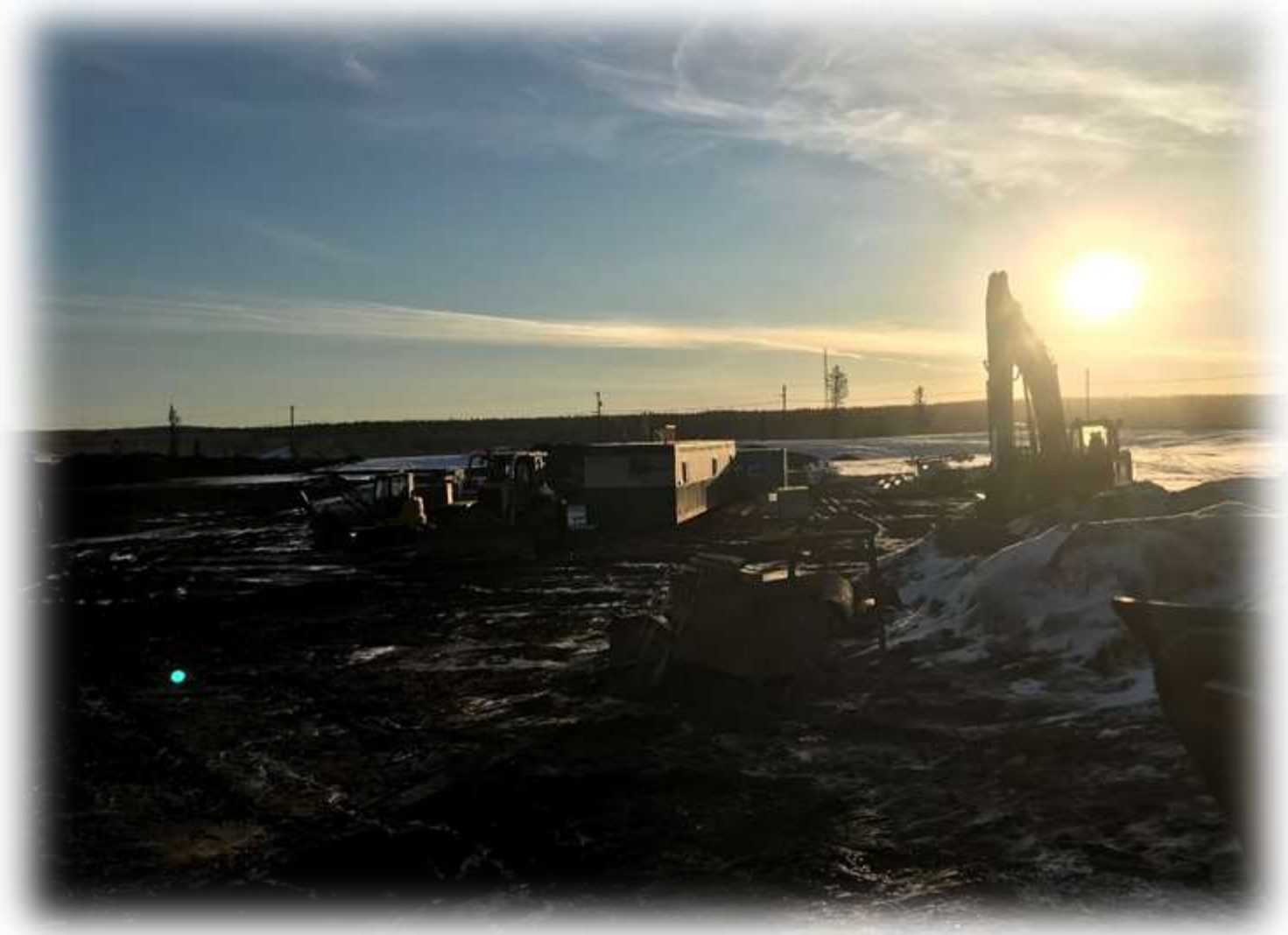
Photos showing Pavilion Laydown Area
