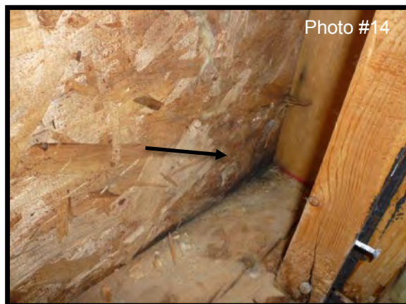
Mould growth was confirmed on the exterior OSB sheathing throughout the perimeter of the facility
