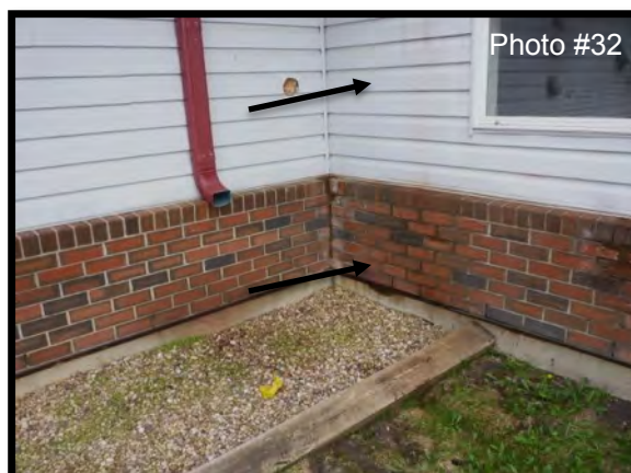
Heavy water staining was noted on the exterior siding and brick cladding in several areas.
