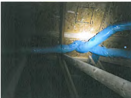
Photo 28: Exhaust ducts terminating at roof vent
