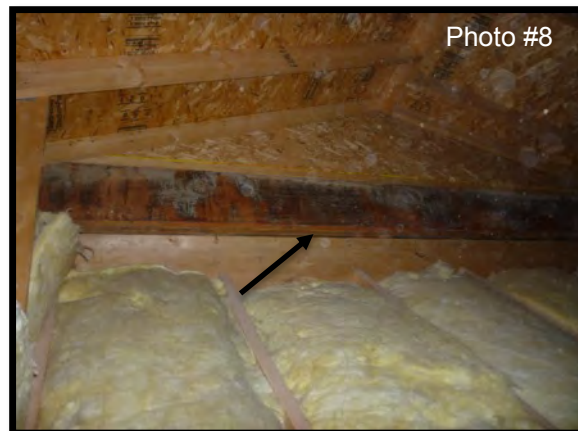
Mould growth was observed on a glulam beam adjacent to the skylight/tower
