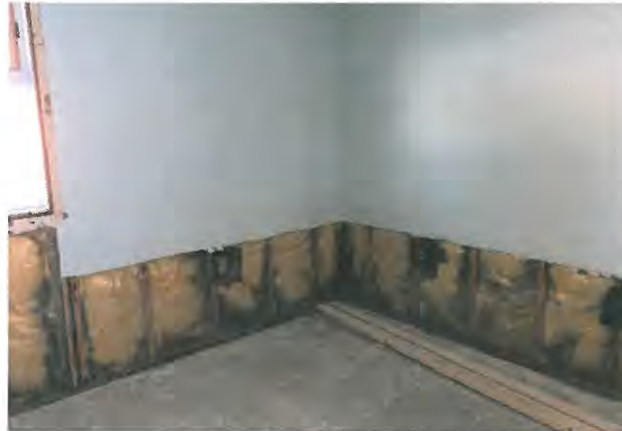
Photo 12: Stained insulation in north office
