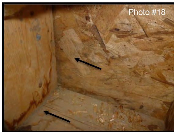
Additional photo showing water stains on a vertical wall stud and fungal amplification on the OSB sheathing
