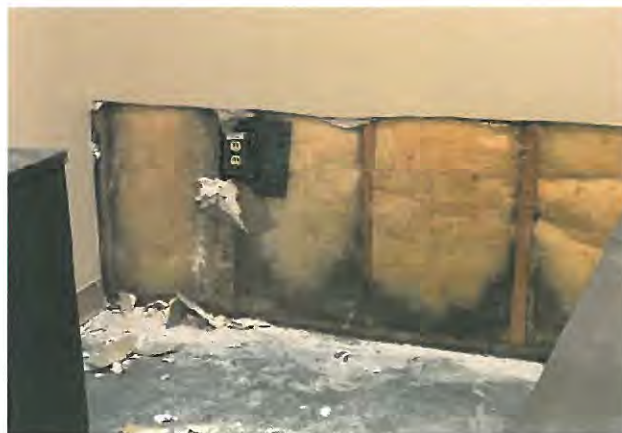
Photo 13: Stained insulation in nurse's office
