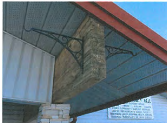
Photo 6: Exposed end of typical glulam beam
