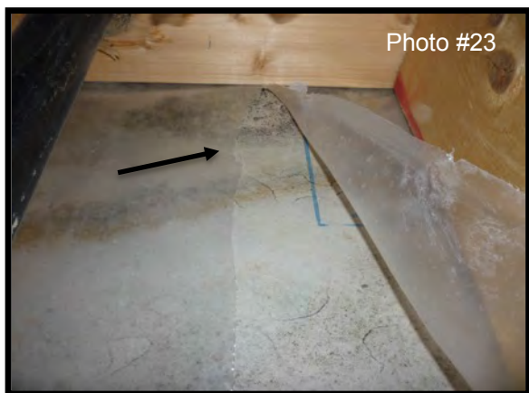
Mould growth on the backside of the drywall within the Men's washroom in the Hall Area
