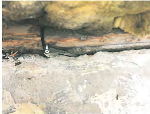
Photo 14: Joint between interior slab and grade beam under typical exterior wall
