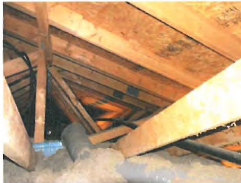
Photo 29: Duct running under insulation across attic floor
