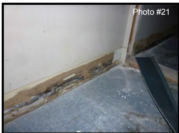
Mould growth was noted on the bottom of the walls in the janitors room (RM 115)
