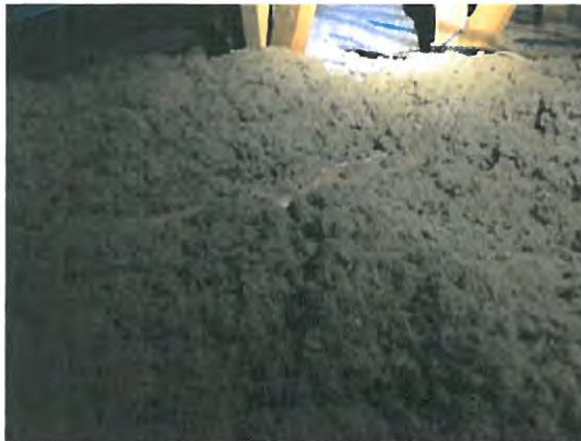
Photo 26: Typical attic insulation cover where insulation appears to have been disturbed
