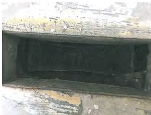
Photo 15: Separated duct at slab penetration
