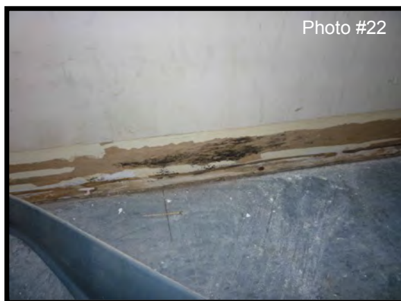
Mould growth was also evident on the bottom of interior walls within the health room, the office bathrooms, and the boardroom
