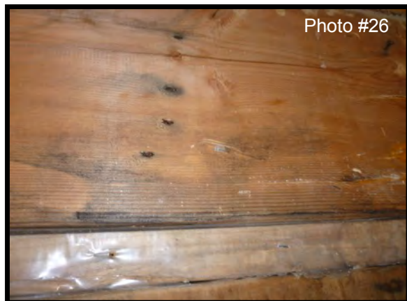
Mould growth on a door header outside Rink Hall Mechanical Room 114
