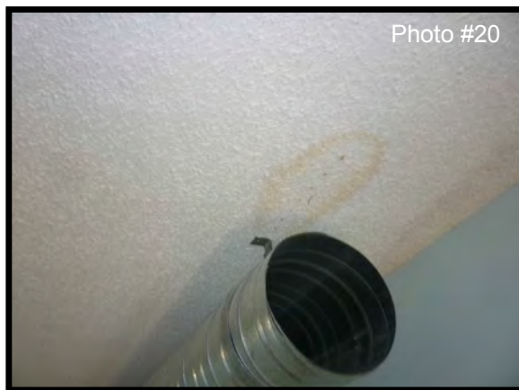
Water staining was also noted on the ceiling in Office RM 124
