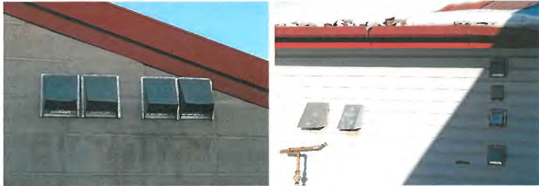
Photos 9 and 10: Reverse lapped vent covers
