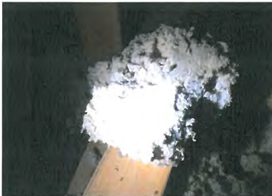
Photo 27: Compressed attic insulation
