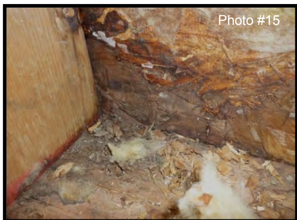
In several areas, the exterior OSB sheathing was heavily damaged
