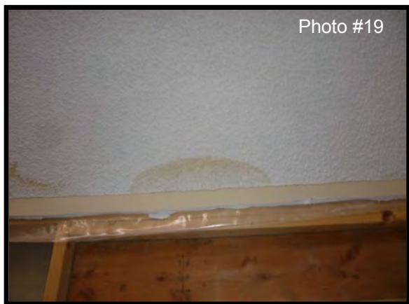
Water staining was observed on the ceiling in the lobby area. Trace amounts of mould growth were confirmed
