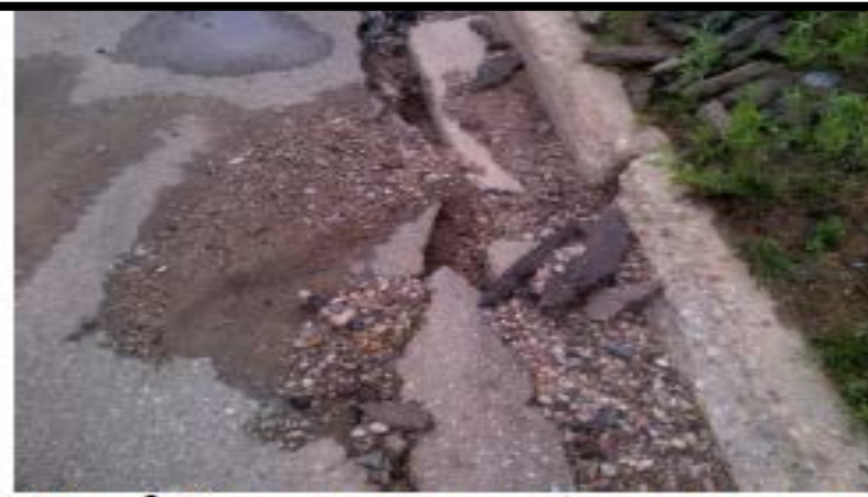
Photo 2: Damage to curb caused by excess pressure
