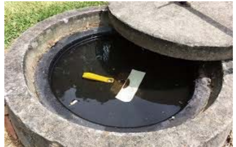
This image shows a manhole insert to prevent river water from entering the system
