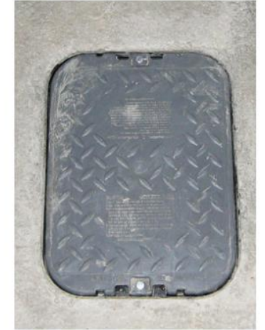
Floor plate cover for backwater valve.
