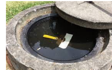
Manhole insert (plug) to prevent river water from entering the system
