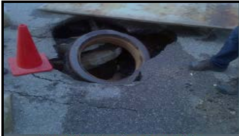
Photo 1: Top view of sunken manhole
