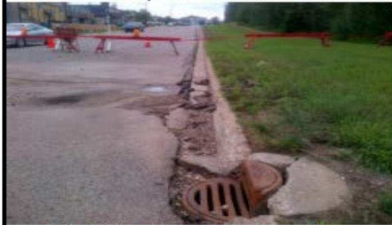
Phot 3: Damage to curb due to overflow
