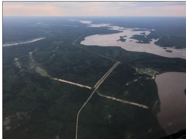
Completed Vegetation Management Areas FB1, 6, 14, & 15
