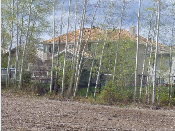
New Combustible Un-Rated Wood Shake Roof – Fort McMurray
