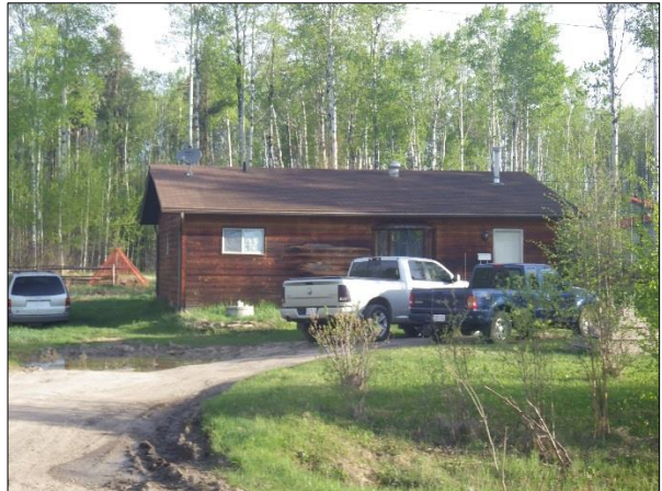
Inadequate Priority Zone Clearance from Surface Fuels
