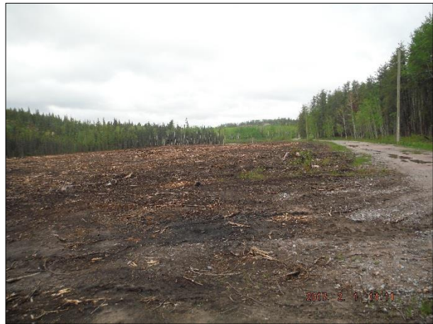
Completed Vegetation Management Area FB3
