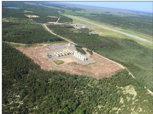
Completed Vegetation Management Area FB5 - Atco Electric Power Station
