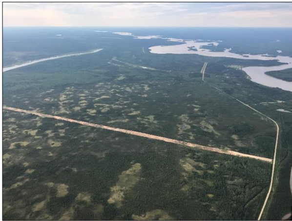
Completed Vegetation Management Area FB13
