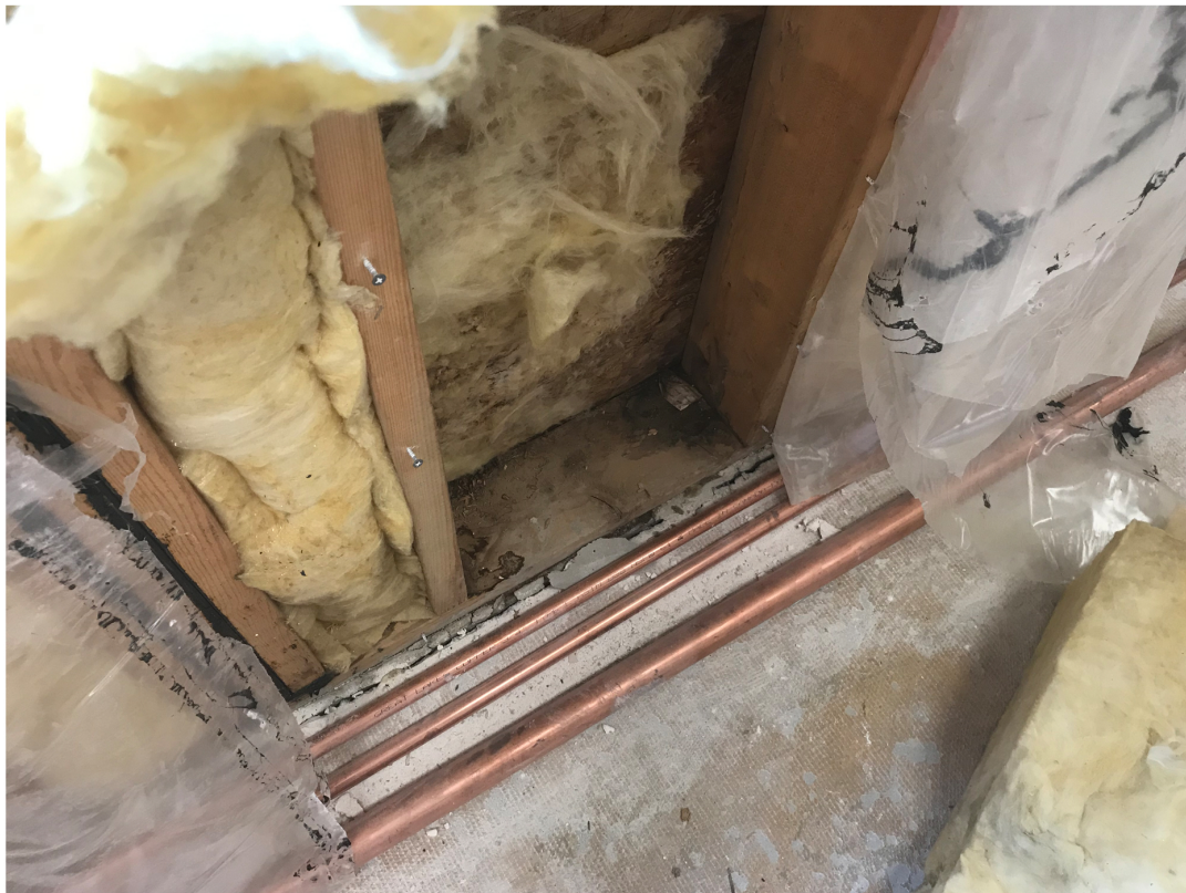
2x6 sill plate in multicultural room before sample taken.JPG
