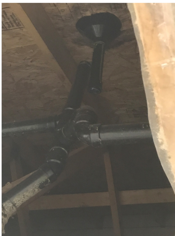
reconnect water vent and replace OSB around top.JPG
