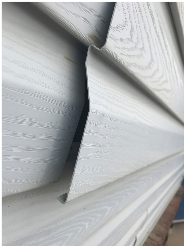
vinyl siding showing some signs of wear in two places on east wall.JPG
