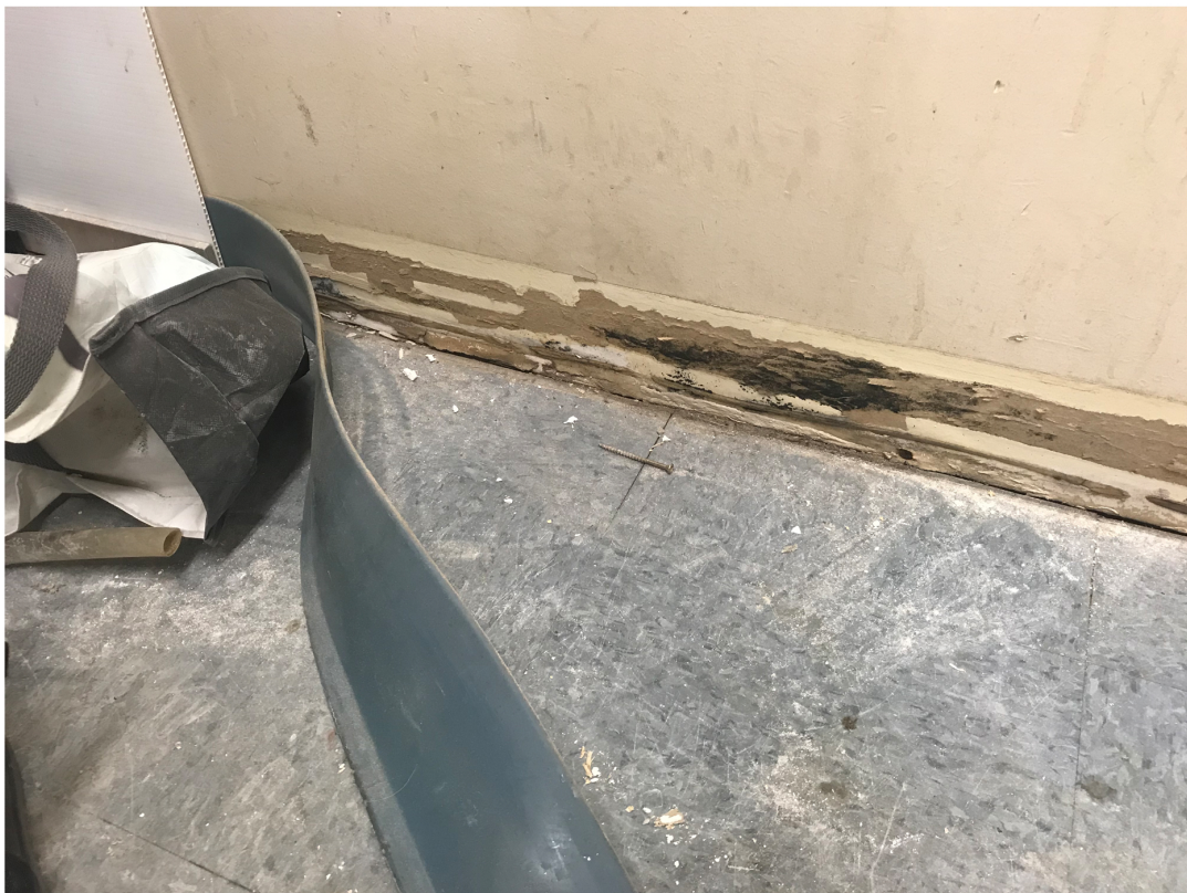
rubberized baseboard in Janitor Room harboured mould growth.JPG
