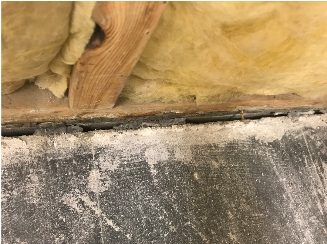
space between floor slab and foundation wall should be filled with epoxy.JPG
