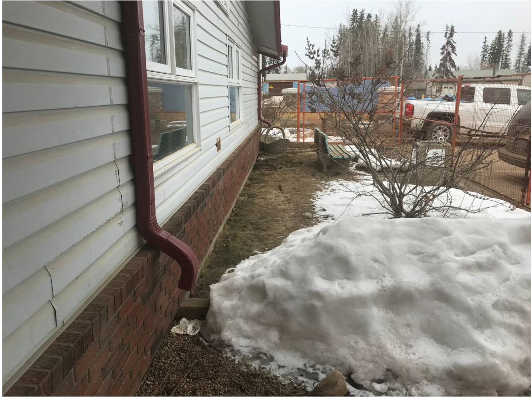
roof downspouts should extend 1.2m away from foundation.JPG
