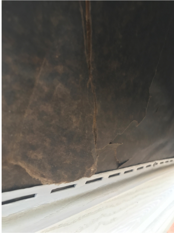
tar or felt paper under vinyl PVC siding showing some wear in a couple spots.JPG
