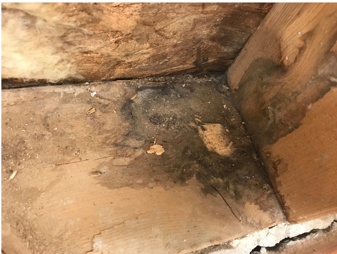
evidence staining on 2x6 sill plate is surficial.JPG
