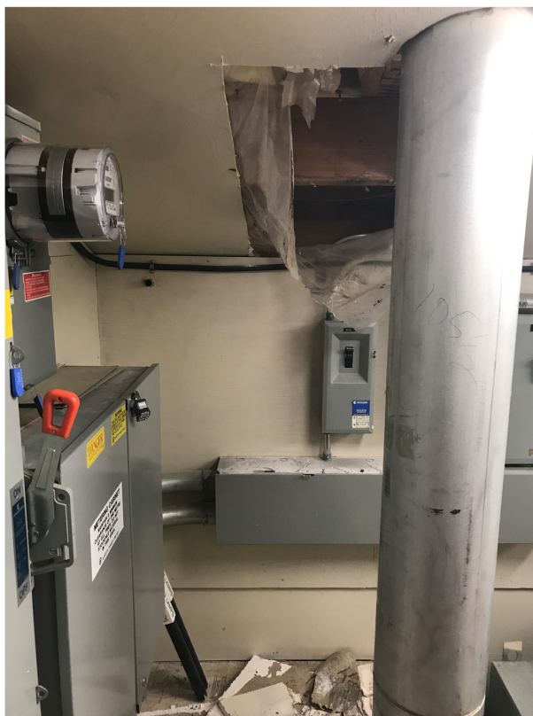
old furnace stack not insulated.JPG
