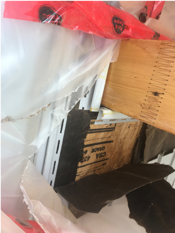
external grade OSB on wall sheeting.JPG
