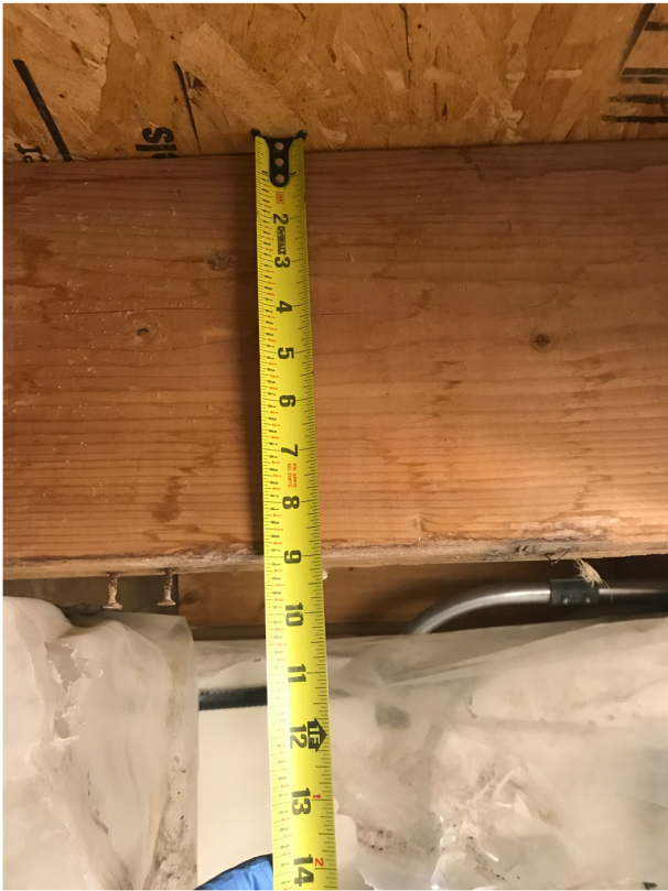
2x10 joists support roof sheathing.JPG
