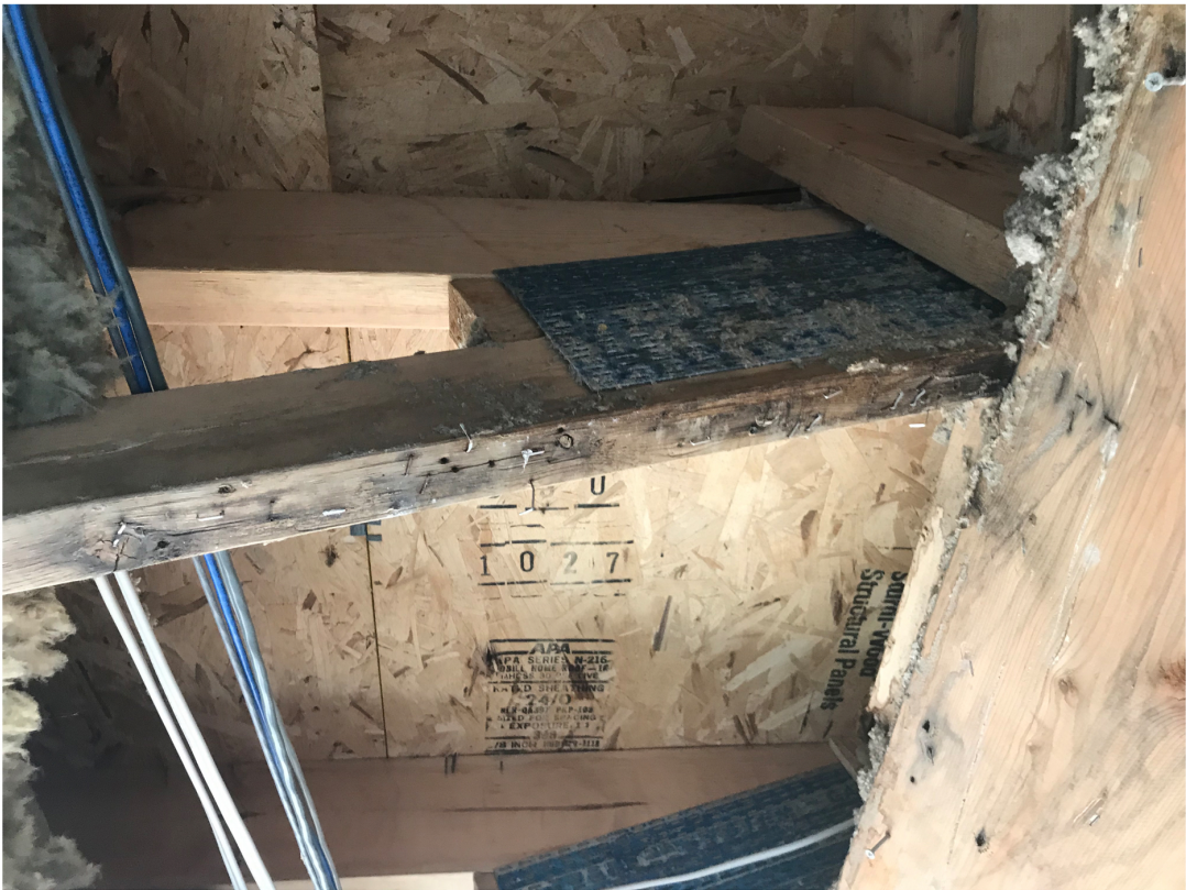
surficial damage to rafters in rink hall.JPG
