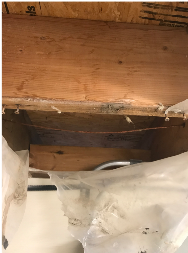
surficial damage in joists below old furnace stack in electrical room..JPG
