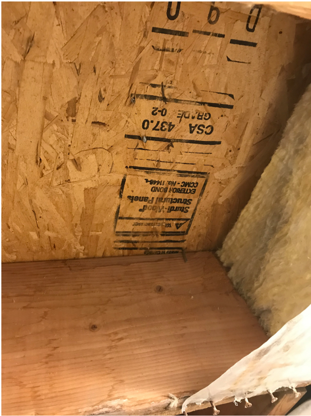
roof sheathing is exterior rated OSB.JPG
