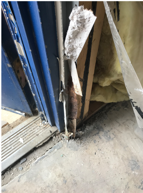
sill under doorway should be sealed with silicone.JPG
