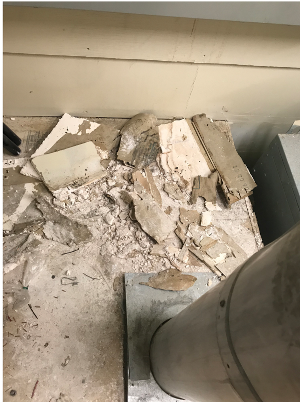
evidence of potential mould in drywall below old furnace stack.JPG
