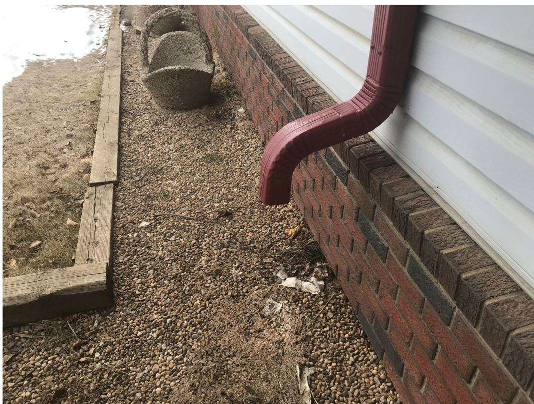
no downspouts extend more than 0.3m from foundation wall.JPG
