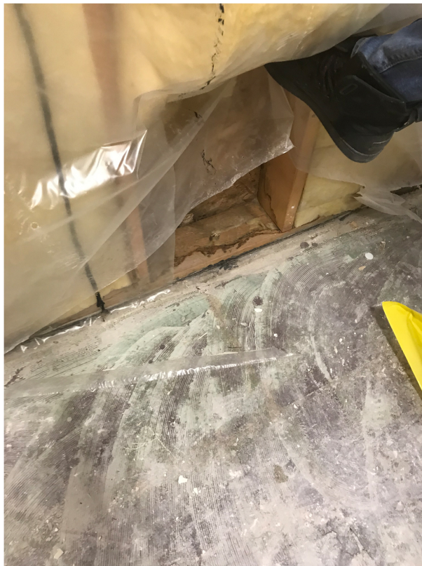
surficial damage to sill plate in change room 1.JPG
