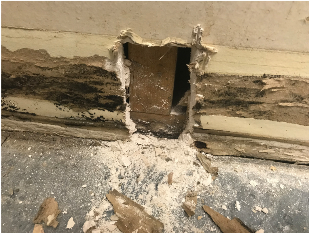
potential mould in janitor room. No damage to studs behind drywall.JPG
