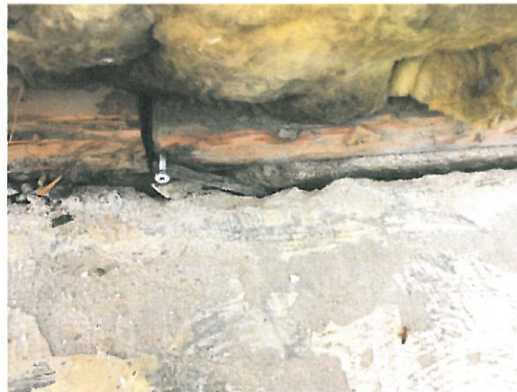
Photo 14: Joint between interior slab and grade beam under typical exterior wall
