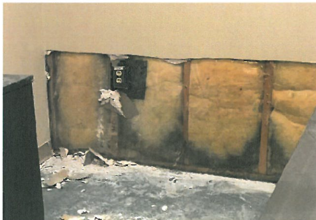
Photo 13: Stained insulation in nurse's office
