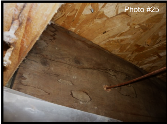
Water staining was observed on a beam in the ceiling cavity above the mezzanine of Mechanical Room 122
