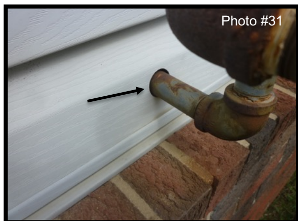
Multiple unsealed penetrations in the exterior siding were noted
