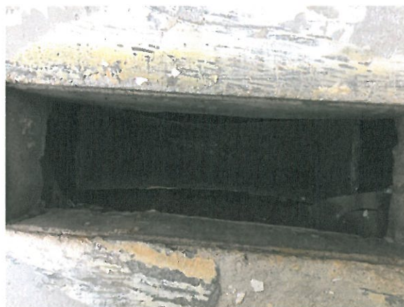
Photo 15: Separated duct at slab penetration
