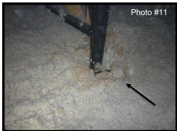
Leakage from around the plumbing stacks had caused water damage and compaction of the attic insulation
