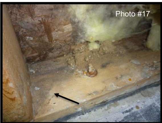
The exterior baseplates had visible water staining and mould growth in several areas
