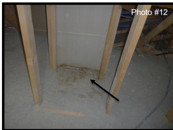
Water stained insulation and drywall within the attic adjacent to the access hatch in Janitor's Room 118
