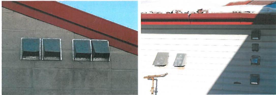
Photos 9 and 10: Reverse lapped vent covers
