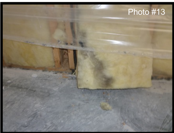
Staining was noted on the exterior wall insulation throughout the facility
