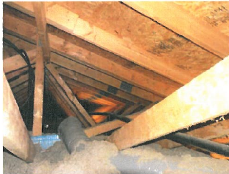
Photo 29: Duct running under insulation across attic floor
