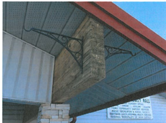
Photo 6: Exposed end of typical glulam beam
