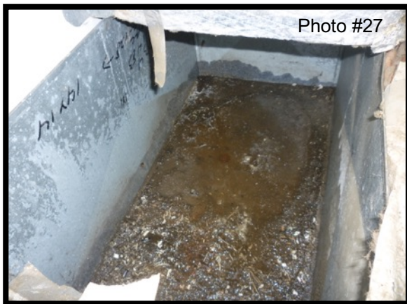
Water pooling and debris were noted in the basin underneath the combustion air duct in Mech. Rm. 114
