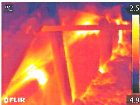
Image 16: Heat loss at top of boardroom wall
