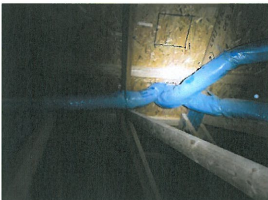
Photo 28: Exhaust ducts terminating at roof vent
