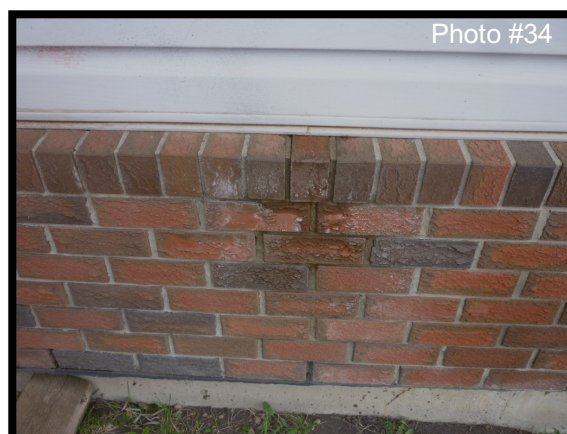
Additional photo showing water staining on the exterior brick cladding
