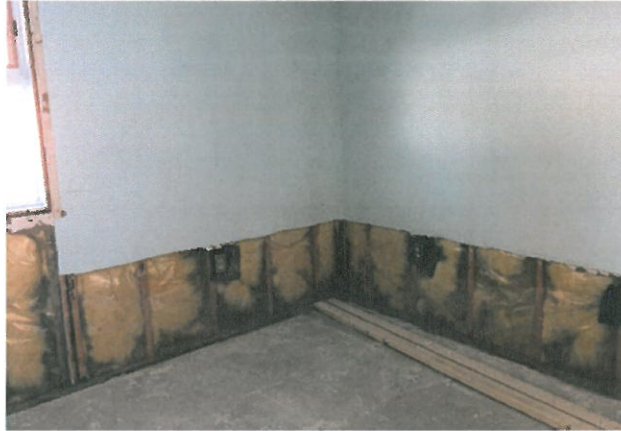
Photo 12: Stained insulation in north office
