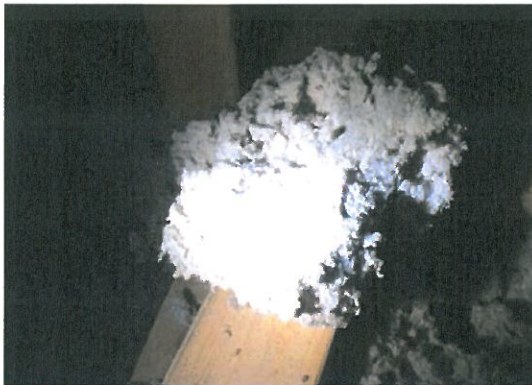
Photo 27: Compressed attic insulation
