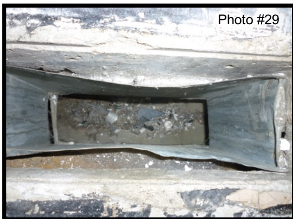
Debris was observed in the in ground supply air ducts. Water pooling inside the ducts is a known concern
