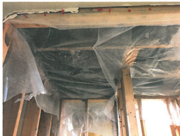
Photo 23: Location of moisture damaged ceiling near Grid D11 per A201
