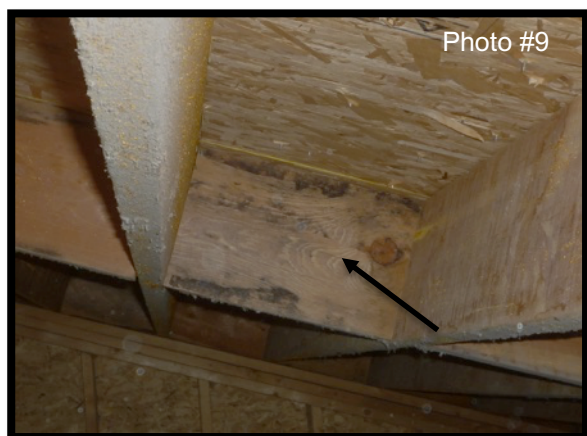
Mould growth was noted on several cross members above the hall area
