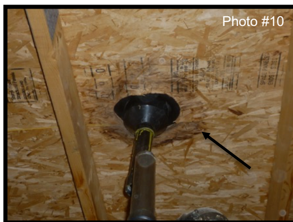
Water damage on the roof sheathing around a plumbing stack situated above the hall area bathrooms
