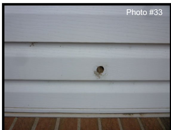
Additional photo showing an unsealed penetration in the exterior siding
